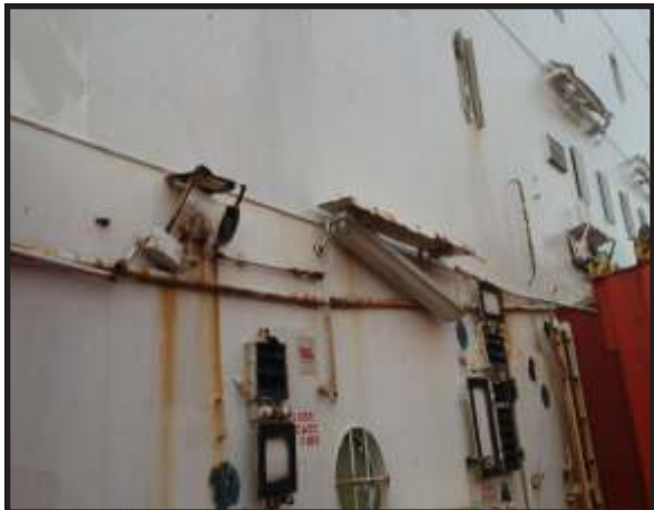
Light shades damaged on decks
